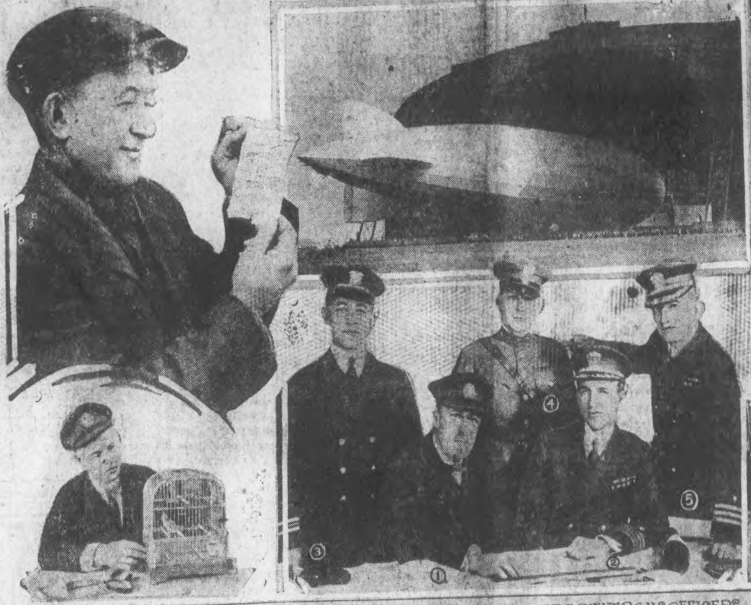
Above: DENNIS SHEA, IN LAKEHURST HANGAR. (Below) CANARY MASCOOT, DR. ECKENER & U.S. OFFICERS. The ZR-3 broke all endurance and distance records when she reached her hangar at Lakehurst, N. J., from Friedrichshafen, a distance of 5,066 miles, in eighty-one hours and seventeen minutes. She is shown here as she is being walked into her hangar. As she passed over New York City, Dr. Eckener, her commander, dropped a message to the press on the International News Service, which was picked up by Jacob R. Klein.
