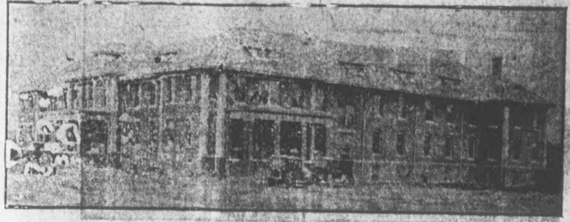
New Dormitory, East Carolina Teachers College, Greenville, N. C.
