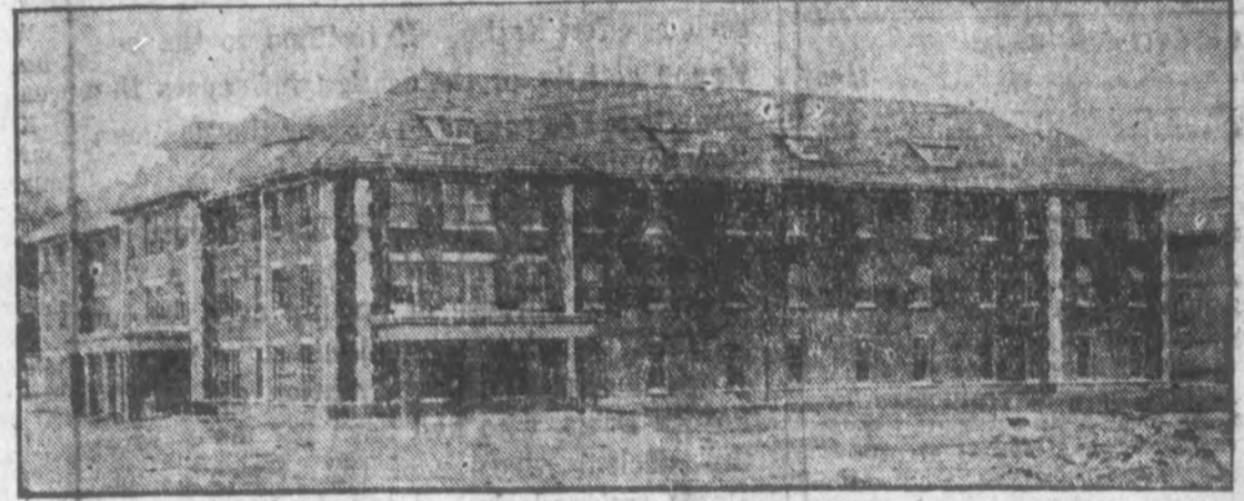
New Dormitory, East Carolina Teachers College, Greenville, N. C.
