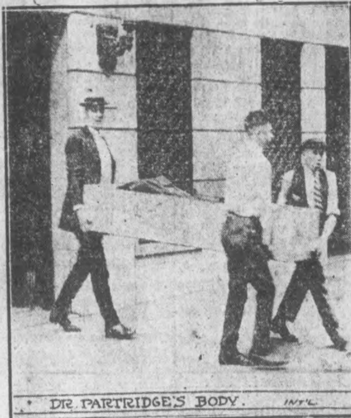
Mrs. James Joughin and Dr. James Partridge were victims when deadly carbon monoxide, seeping into their New York apartments from a leaky furnace, suffocated them. Photograph shows Dr. Partridge's body being carried from the building where he lived.
