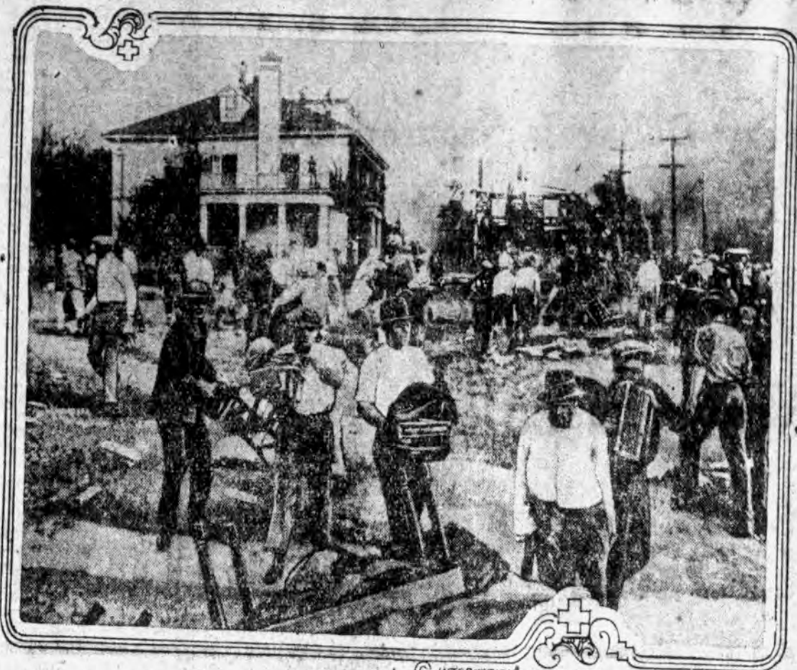
SAVING PROPERTY ON THE EDGE OF A GREAT FIRE WHILE RED CROSS WORKERS SERVE THE INJURED AND HOMELESS
