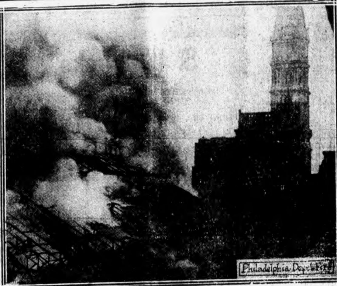
Here is a striking picture of the $5,000,000 fire which destroyed the Broad Street Station of the Pennsylvania Railroad, in the heart of Philadelphia, imperiling many passengers. In the right background may be seen the Philadelphia City Hall, one of the finest public buildings in America, which for a time was thought to be in danger of destruction.
