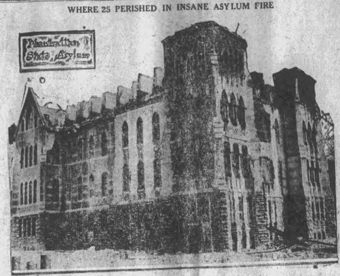
This is the exterior of the antiquated four-story building, one of the group in the Manhattan State Hospital for the insane on Ward's Island in Hell Gate, East River, New York City, where 22 insane patients and three attendants perished in a fire which swept the structure. The roof caved in on them.
