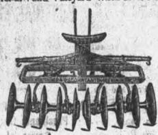
It has a low frame, which will clear overhanging branches and vines. The gangs can be set close together or graduated at intervals of two inches until they spread to their extreme width on the ends of the frame.
