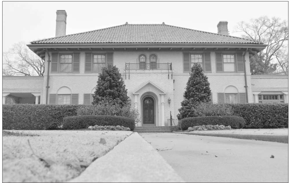
The Dail House is the traditional home of ECU's chancellor, but requires renovations to be usable.
