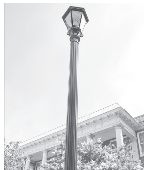
Existing light fixtures also received an upgrade. MIKE SEEGARS | THE EAST CAROLINIAN
