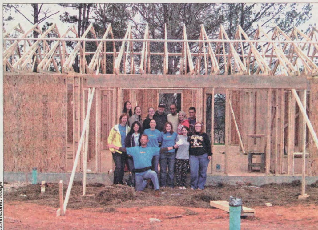
Alternative Spring Break participants stand in front of the finished frame of a house built on the trip.
