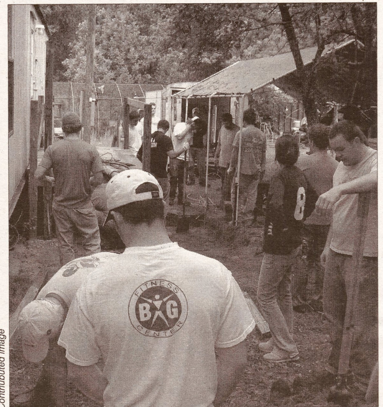
Construction management students help build local woman a wheel chair ramp.
