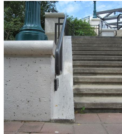
Example of a Flat-Style Stair Channel Lafayette, IN
