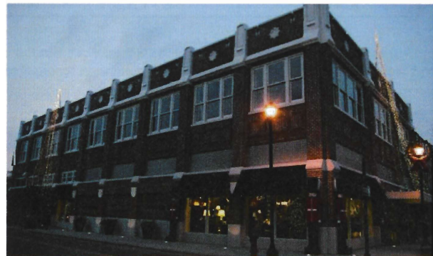
Blount Harvey Building in Greenville
