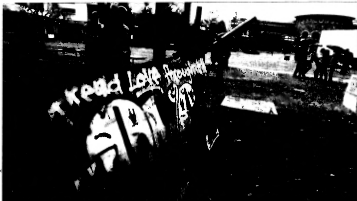
To wrap up Hate Out Week events last week, the wall containing racial slurs and words of hate was demolished.
