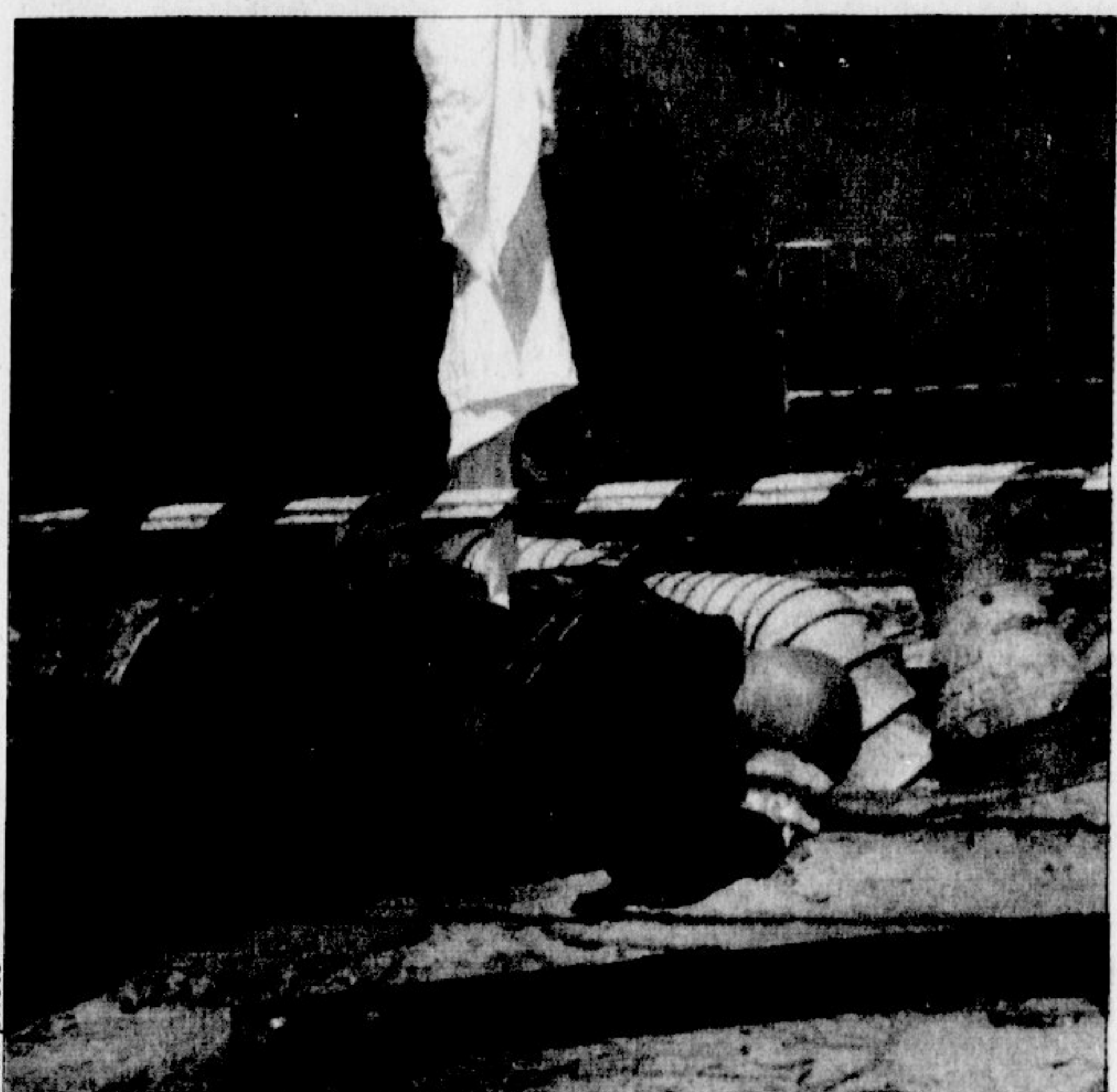
Facility personnel alternate turns working in the manhole to patch a hole within a heating system pipeline.
