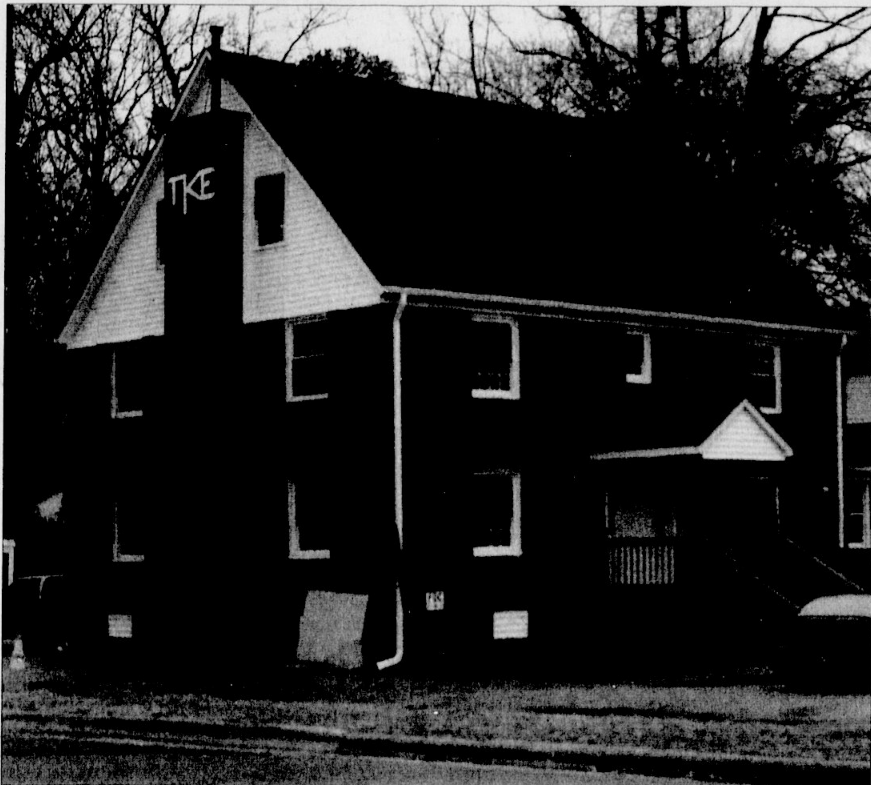
Tau Kappa Epsilon completed their renovation and is now the first Greek house on ECU's campus to have a sprinkler system as a fire safety measure.
