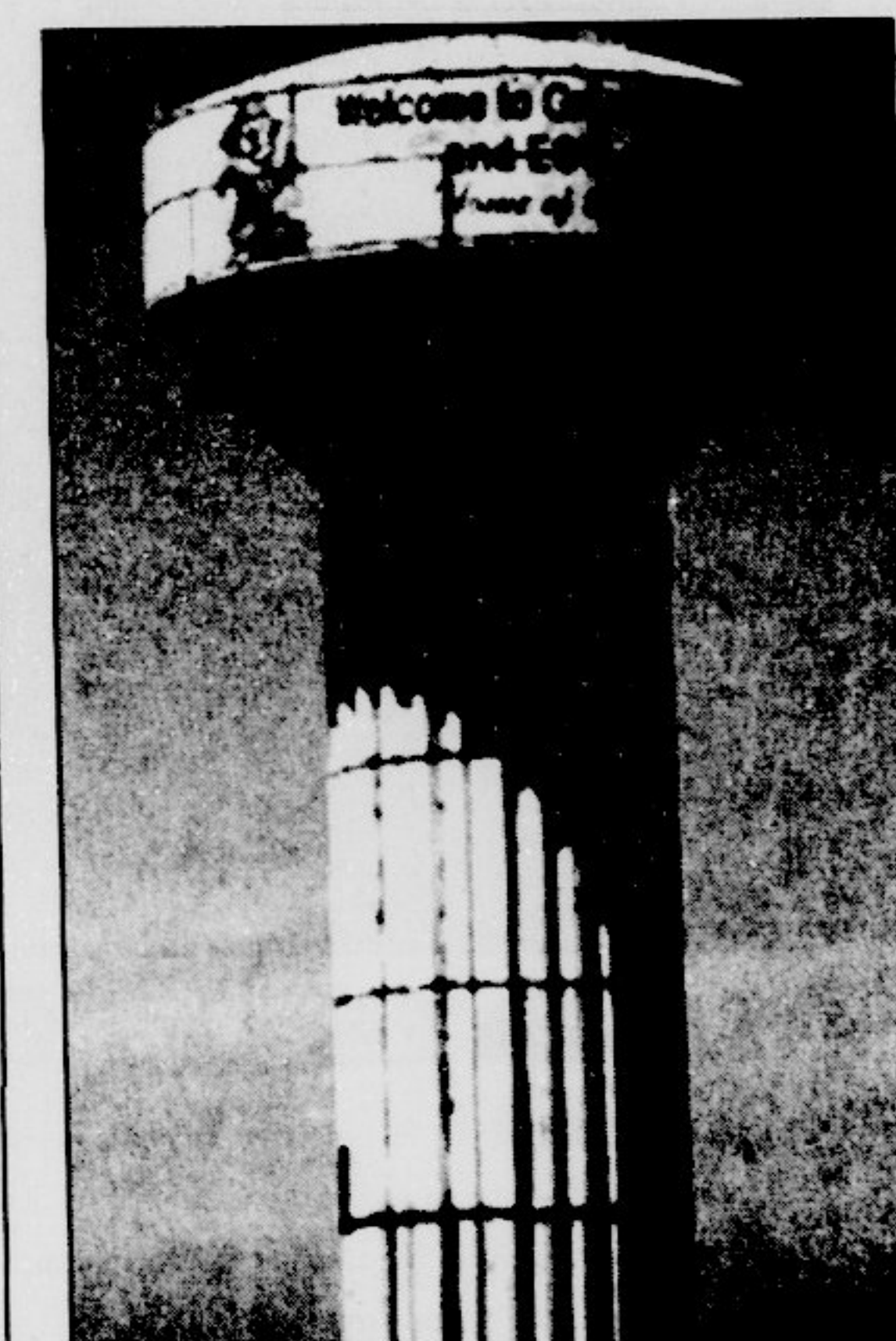
Everyday, total strangers from miles away gaze at one of Greenville's and ECU's proudest symbols. When the city received a new water tower, the old one went into storage. Now the old tower has been resurrected in Columbia, MS which is located 30 miles west of Hattiesburg. PHOTO COURTESY DON LAWRENCE HERITAGE JEWELRY, COLUMBIA MS
