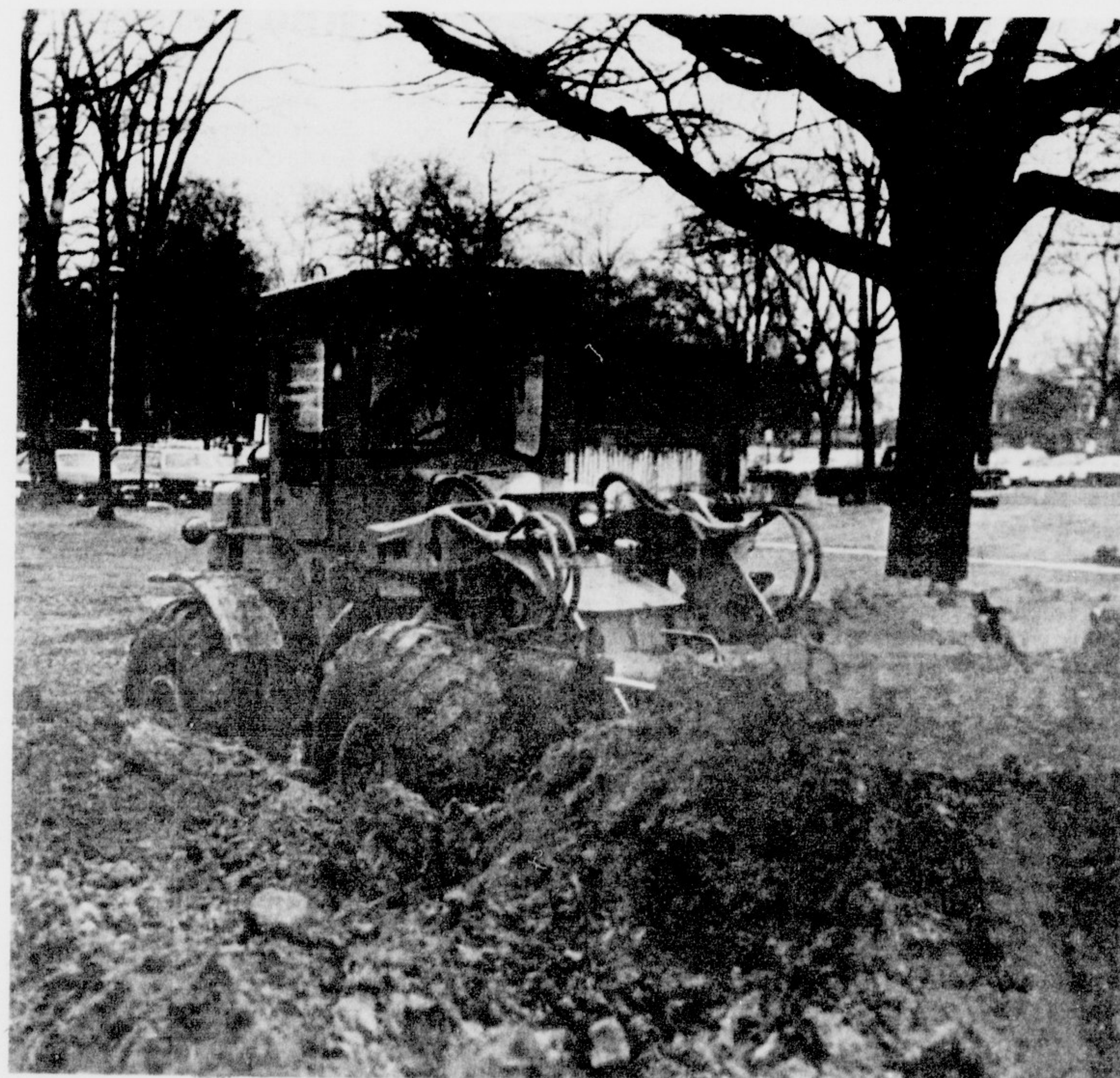
ONE STAGE of this drainage project nears completion.
