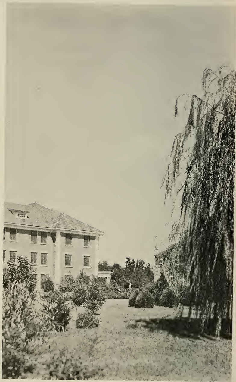
COTTEN HALL AND CORNER OF THE ADMINISTRATION BUILDING ACROSS WRIGHT CIRCLE
