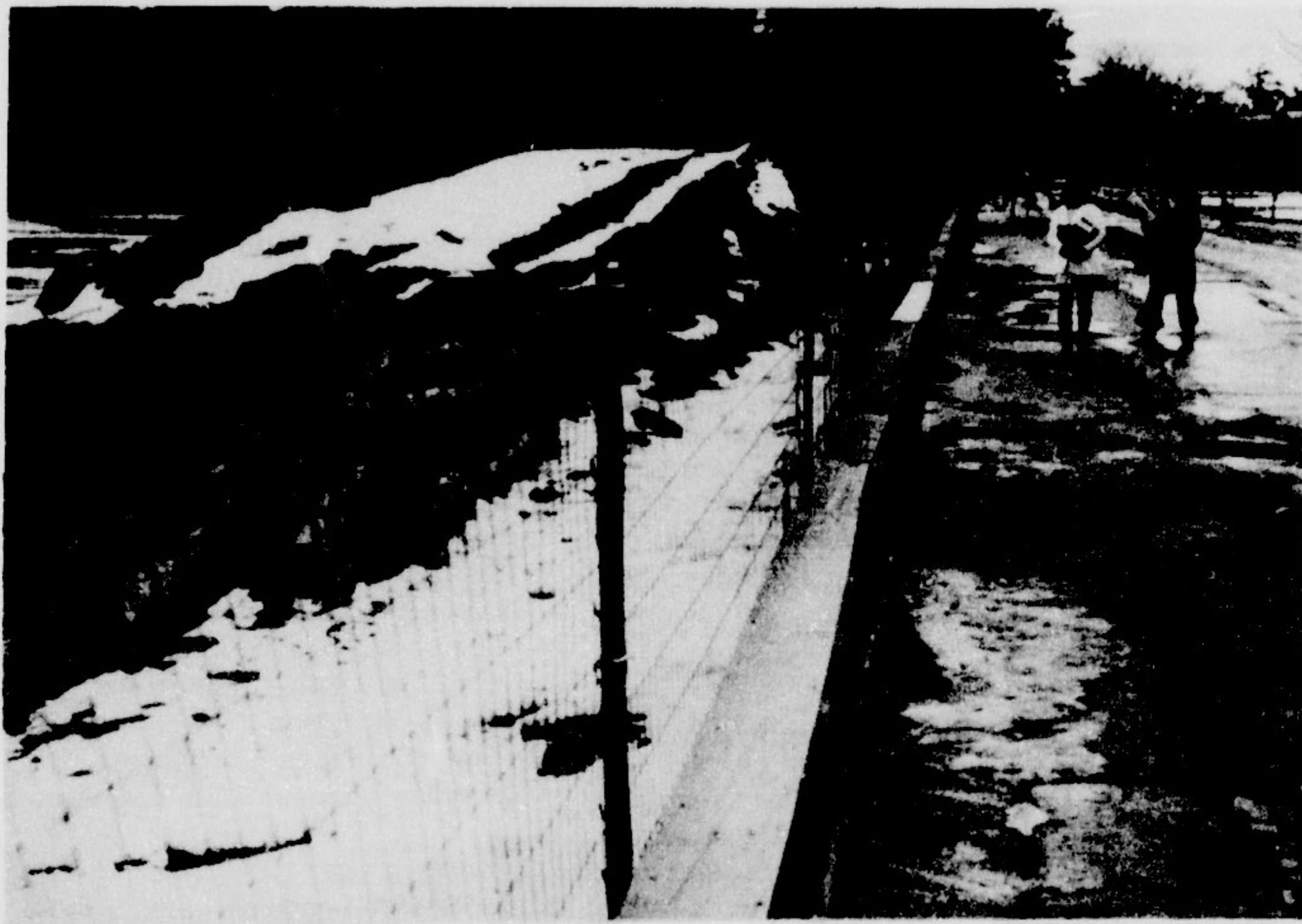
STUDENTS SKIRT the edges of the Art building construction near Jarvis
