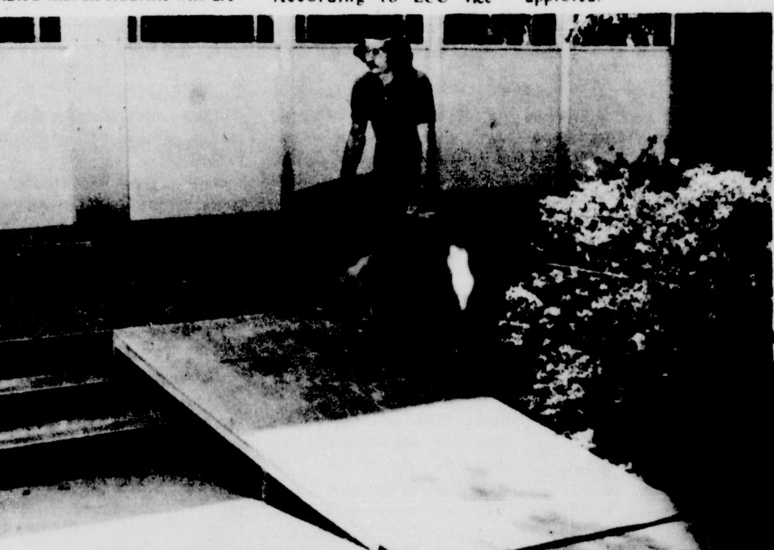
THE BARRIER-FREE PROGRAM to be initiated at ECU this fall will include some 70 ramps to provide easy wheelchair movement around campus. The barrier-free condition at ECU is being made possible by a grant from the N.C. Department of Vocational Rehabilitation with 20 percent matching funds from ECU.
