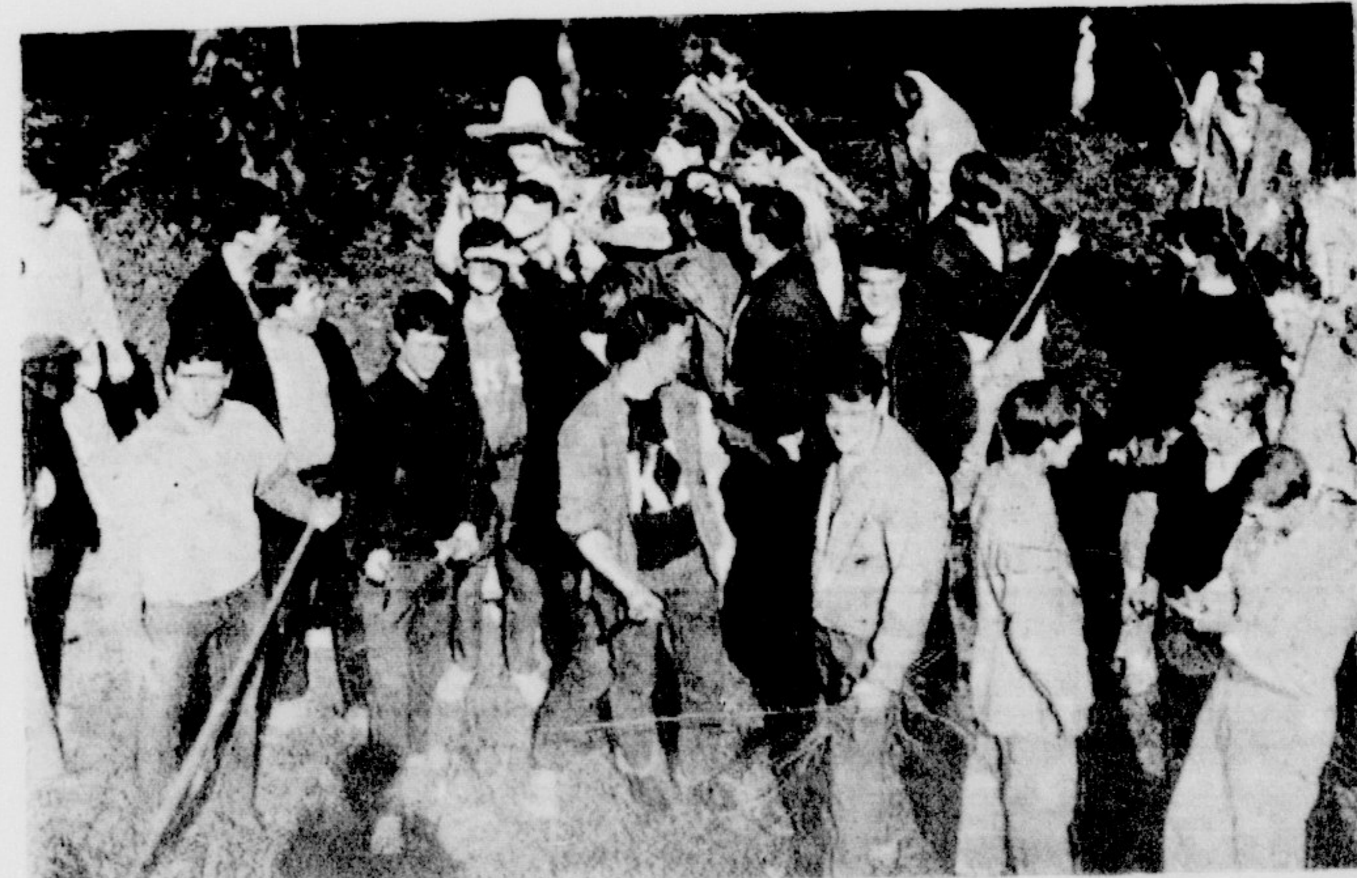
IFC WORK—Members of the Inter-Fraternity Council work on the new park on the east end of Greenville, as they do clean-up behind the heavy equipment. The IFC has taken this work as a special project.
