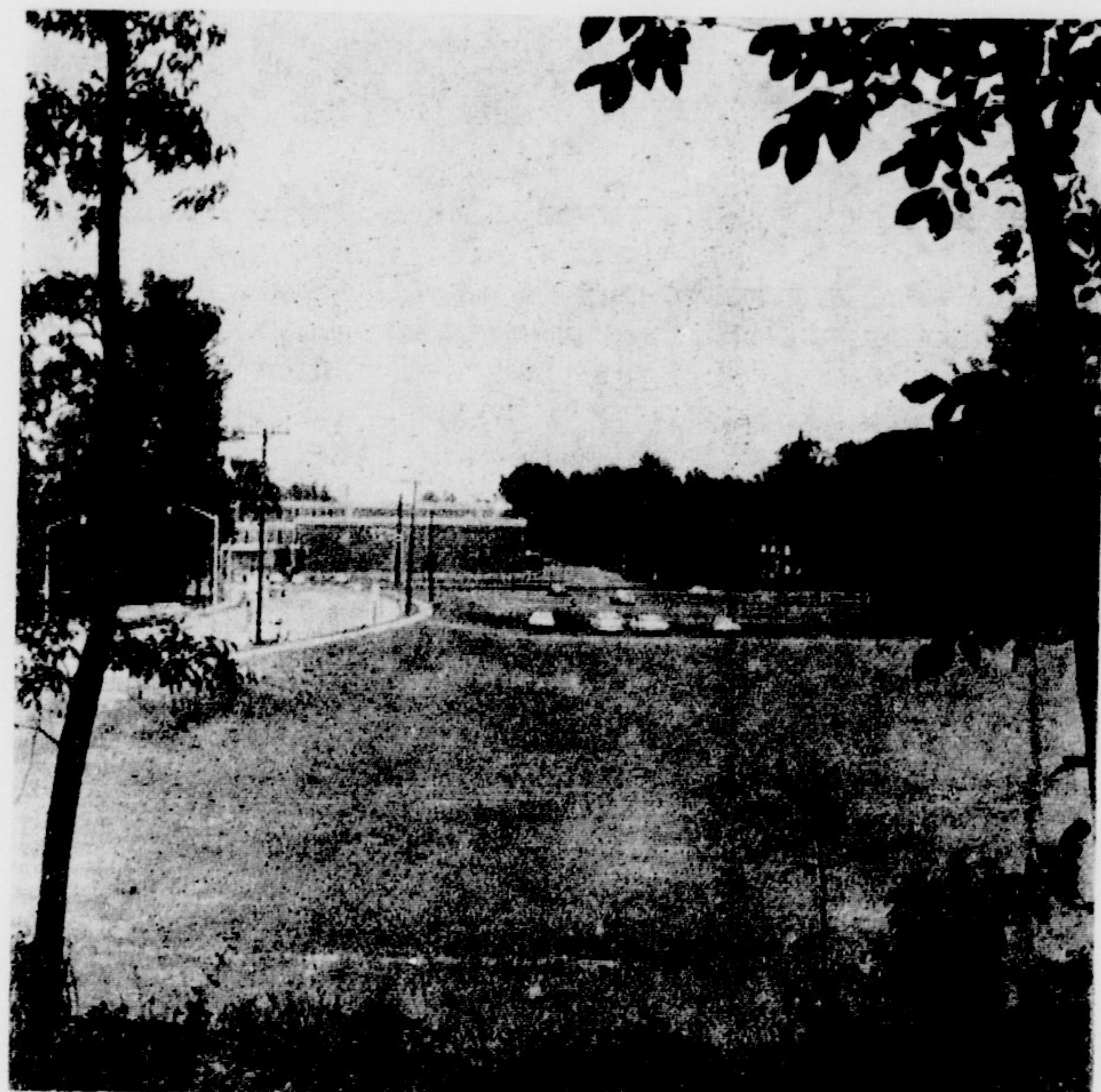
NEW PARKING FACILITY—Construction is soon to begin on this quiet area between Jones Hall and Tenth Street, as bulldozers and other heavy equipment move in to build another day student parking lot. When finished, the lot will hold 250 cars and will bring the total on-campus parking spaces to 2,700.
