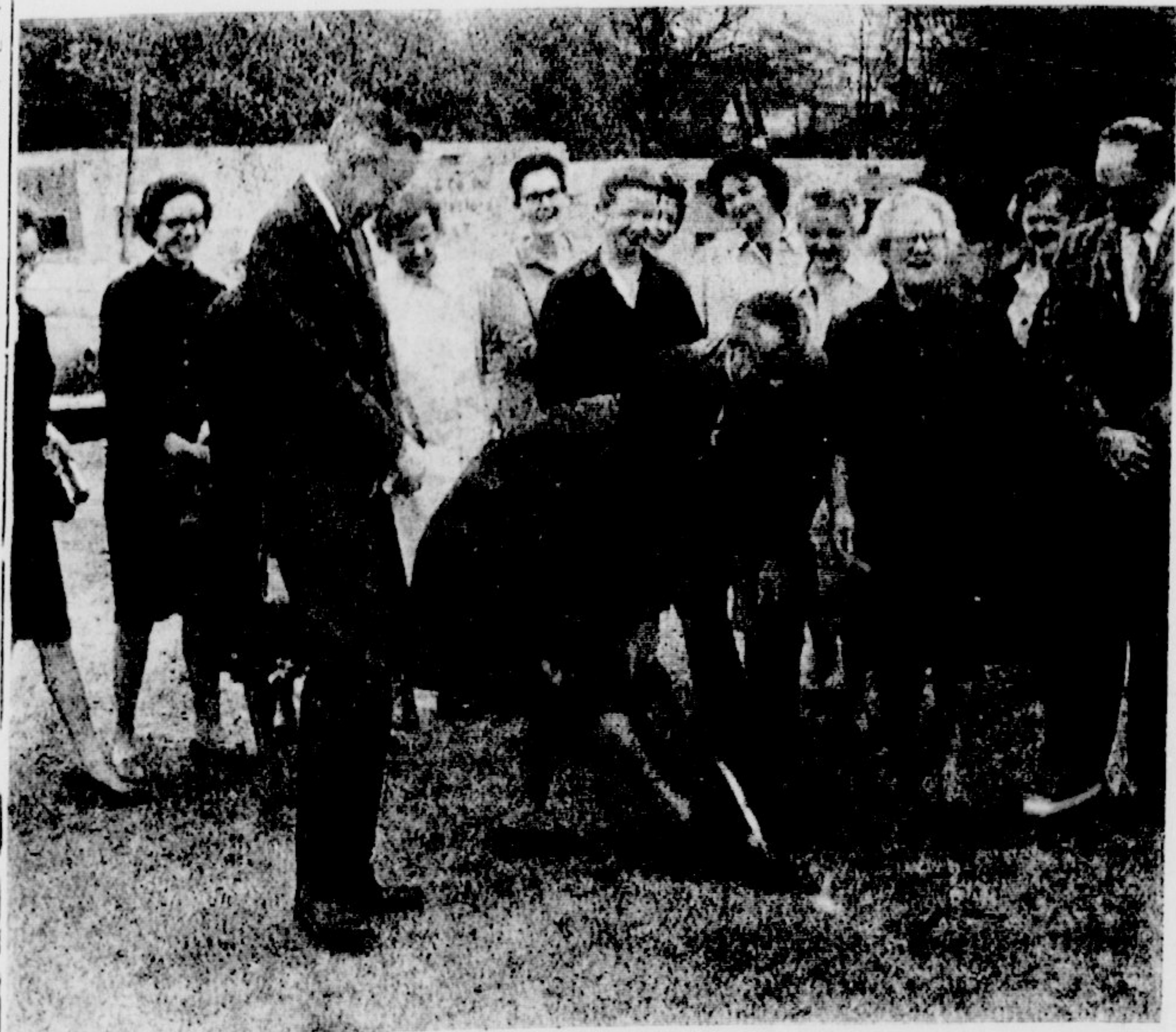
HISTORICAL SPADE—Ground breaking ceremonies for the new School of Nursing were held last week as the traditional Jarvis Spade once again turned the first earth for construction.
