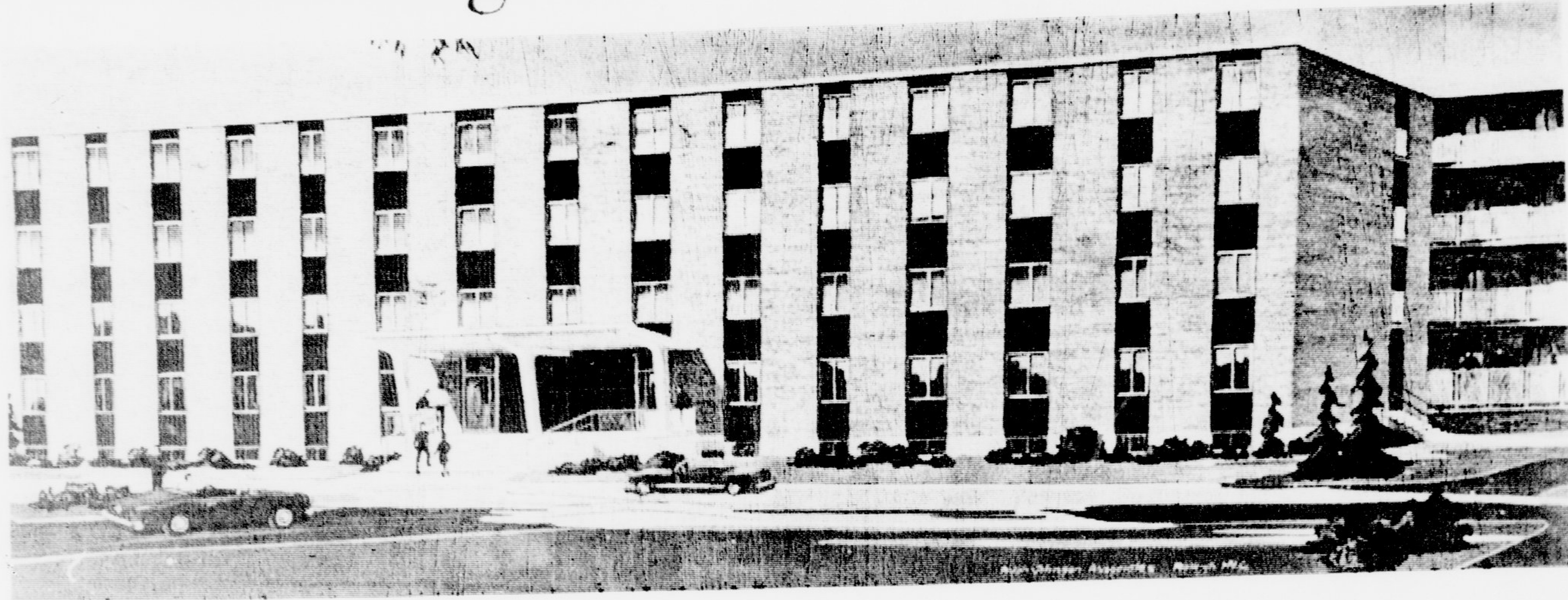
This new men's dormitory, being constructed at the end of College Hill Drive, will house over five hundred men students when completed in July of 1966. The structure will be the fourth dormitory to be built on College Hill Drive since 1959. When it is completed, the complex will house over one thousand men.
