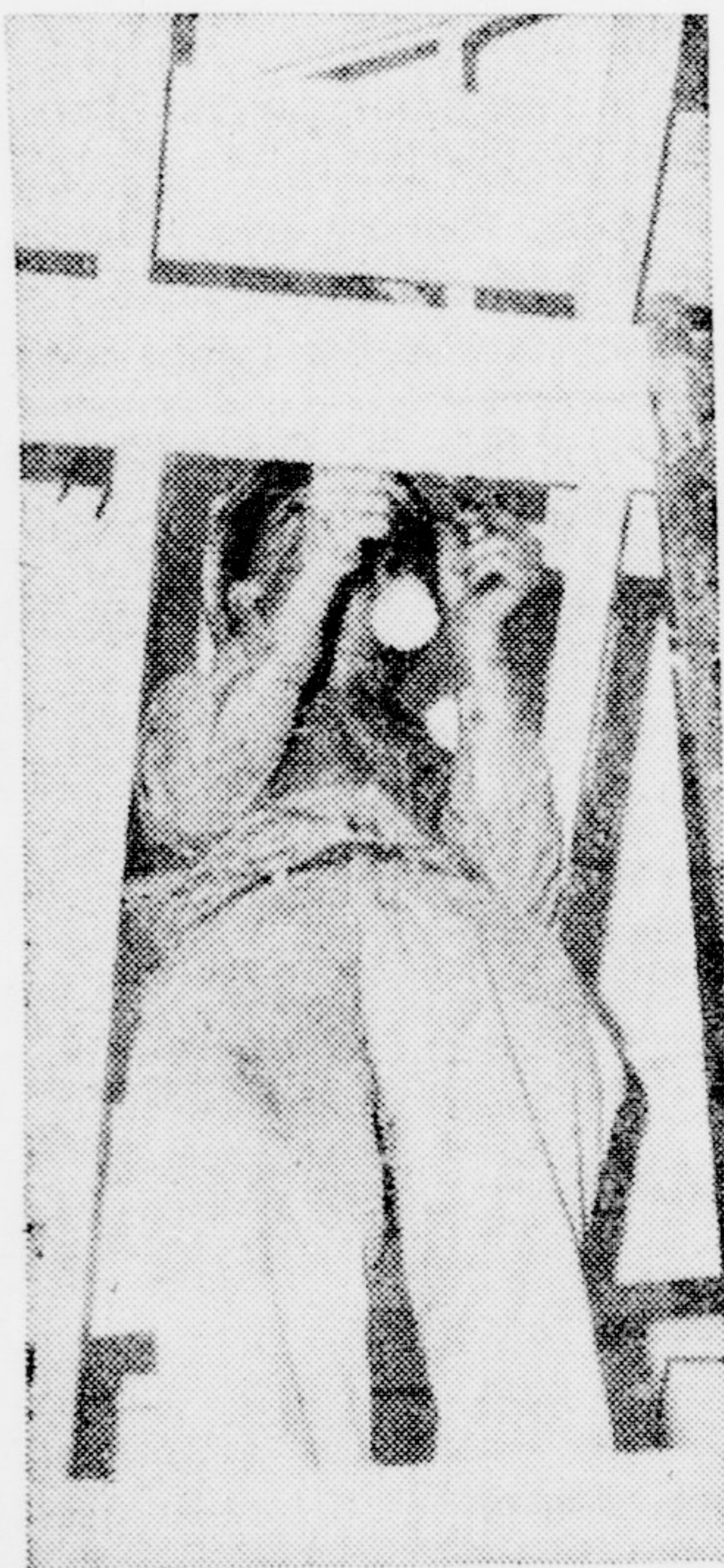
An electrician works in Wahl-Coates Elementary School.
