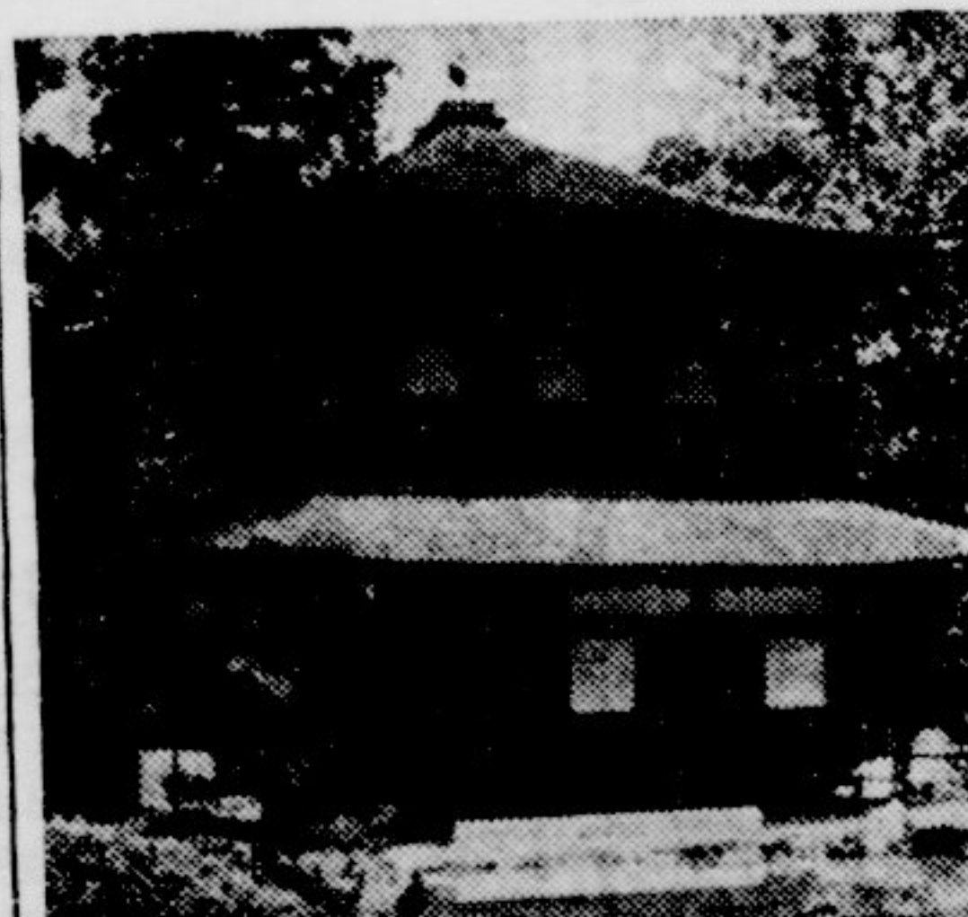
TEAHOUSE . . . Buildings of this type are numerous in Japan.
