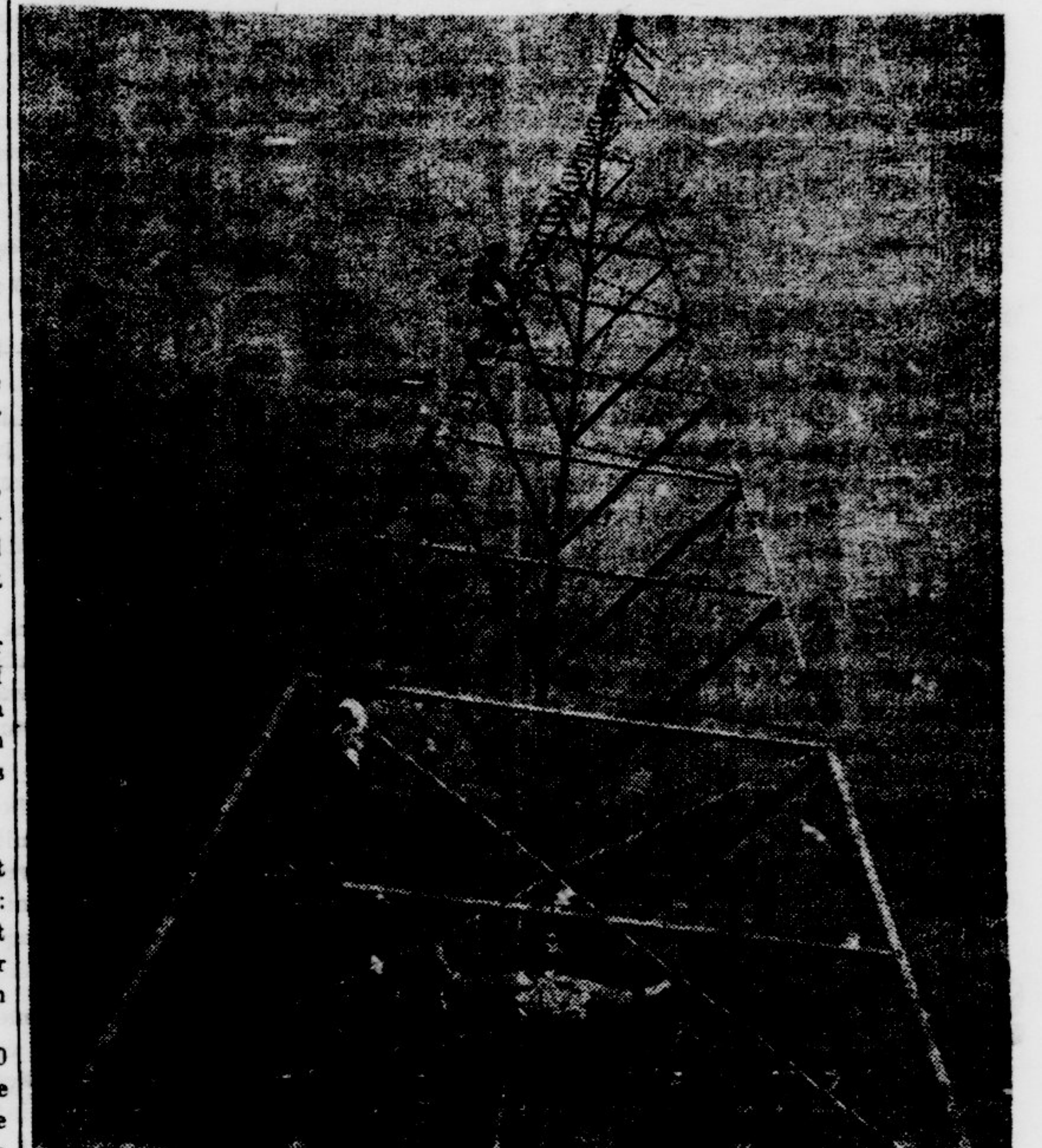
As the huge 135-foot radio tower was being erected atop Joyner Library this week, all technical problems concerning East Carolina's FM radio station were nearing completion. Officials say operation should begin around the first of the year. (Nora Willis photo)
