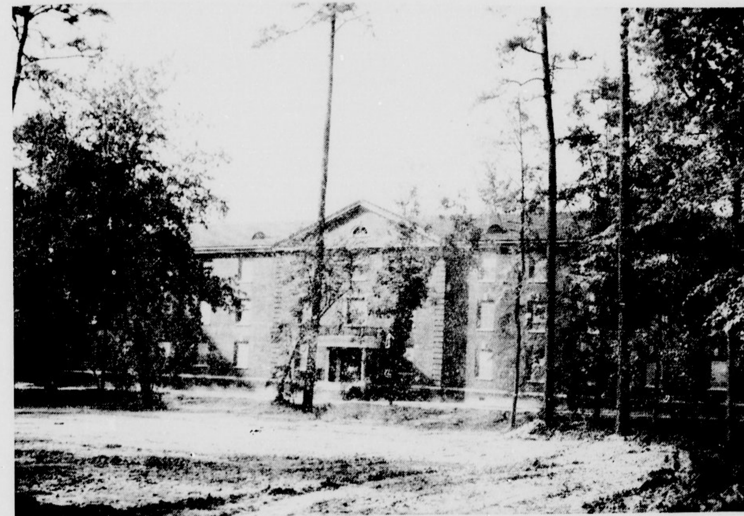
Here is a view of Slay hall, a dormitory for East Carolina men completed this summer. The modern, spacious building has accommodations for 216 persons. It was first opened to students at the beginning of the second summer term.
