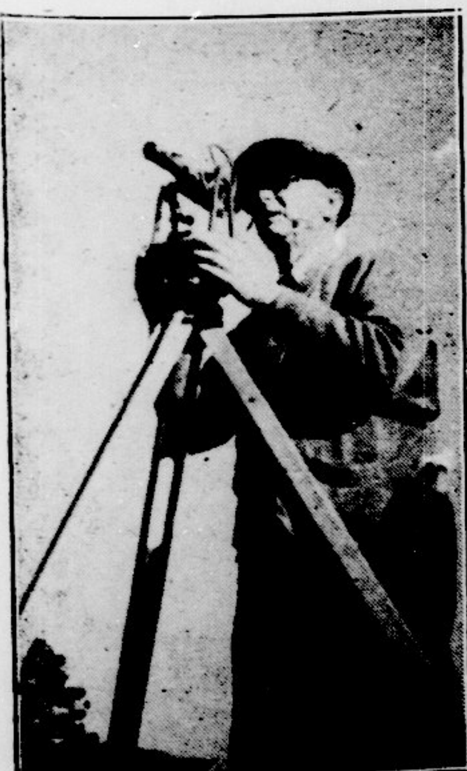
The surveyor pictured above is shown laying off boundaries preliminary to beginning excavations on the new Classroom Building last year. On the right above is a picture of a steam shovel, "machine labor," in operation, making excavations last year as a preliminary step in the construction of the new building.
