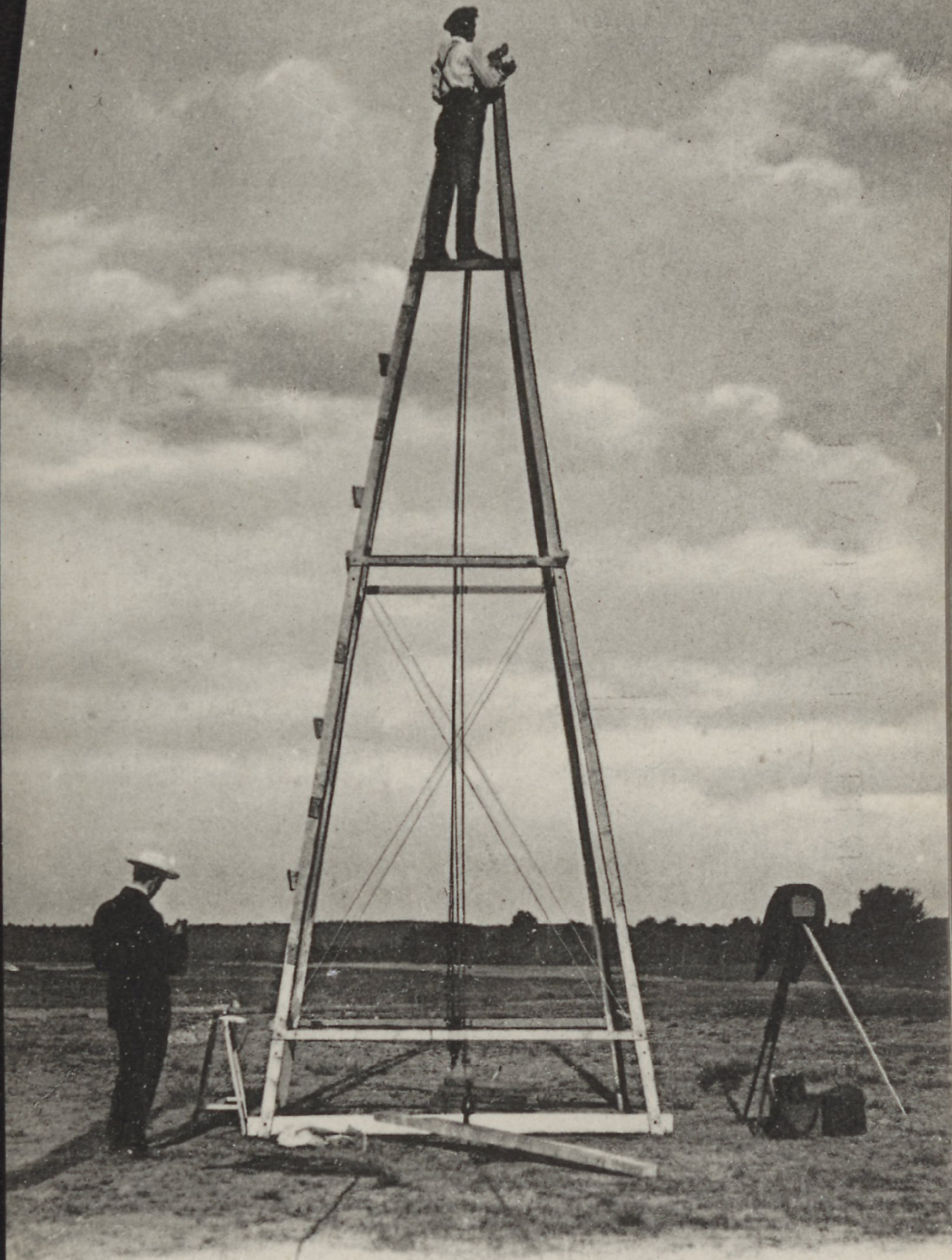
12 Installation du pylône de lancement Installation of the starting ground
