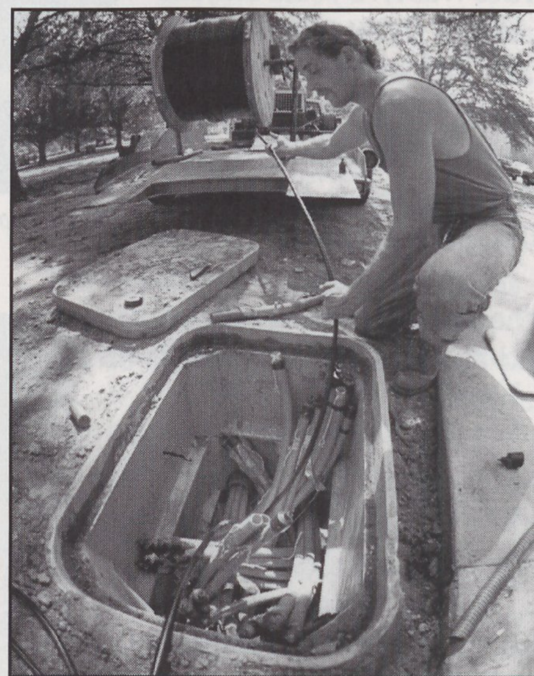
Installing ECU's fiber optic network.
