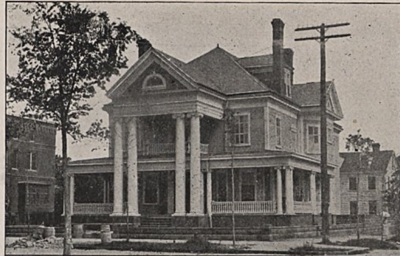
Residence of L. H. Vollers; H. E. Bonitz, Architect; Joe Schand, Builder.
