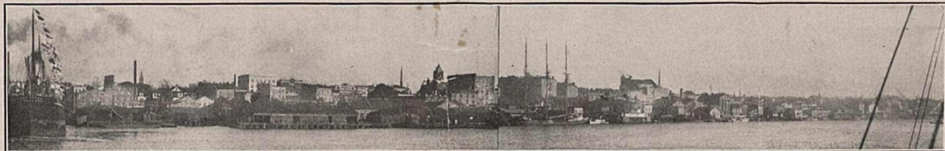
Wilmington's Water Front.
