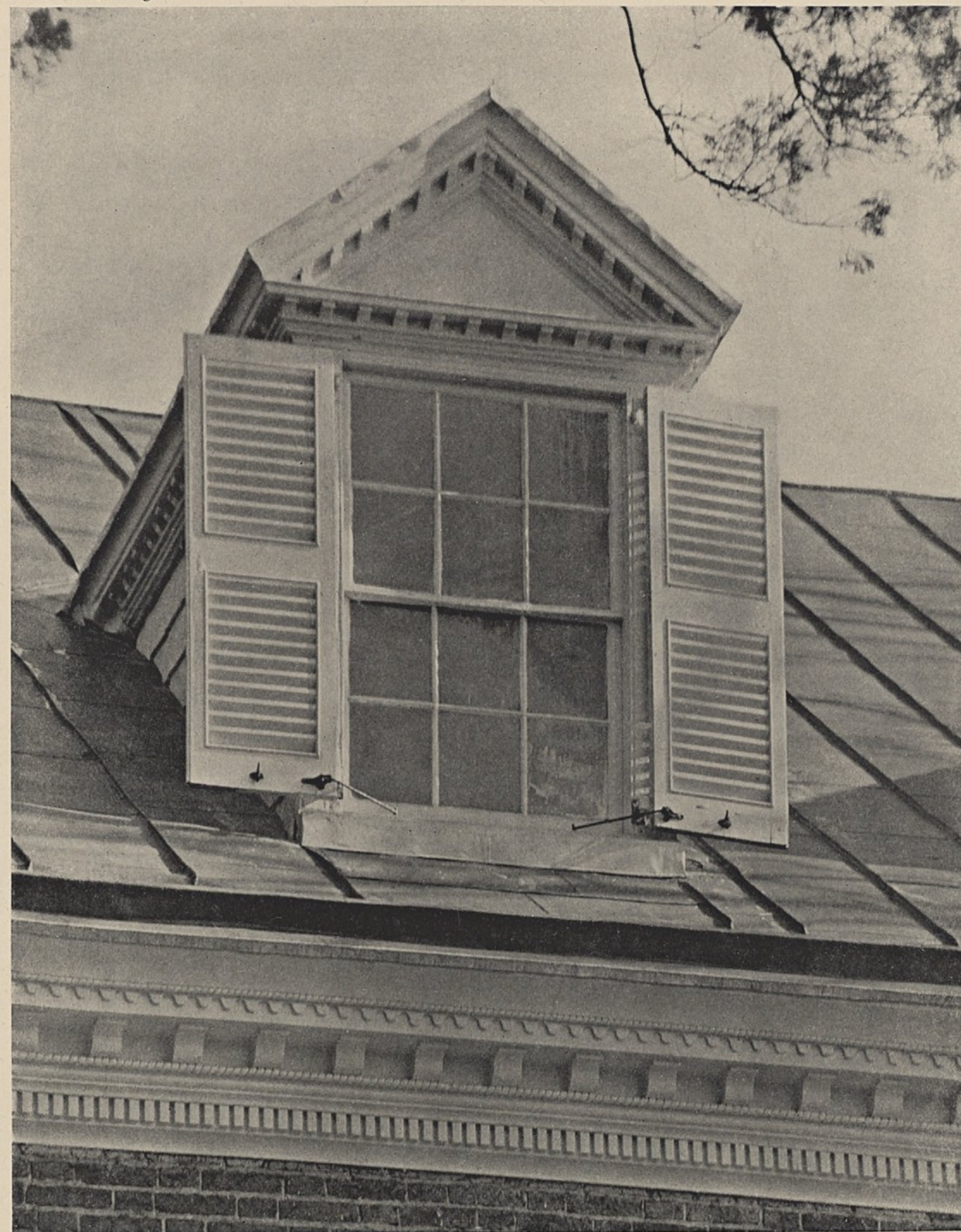
Detail of Dormer and Cornice
