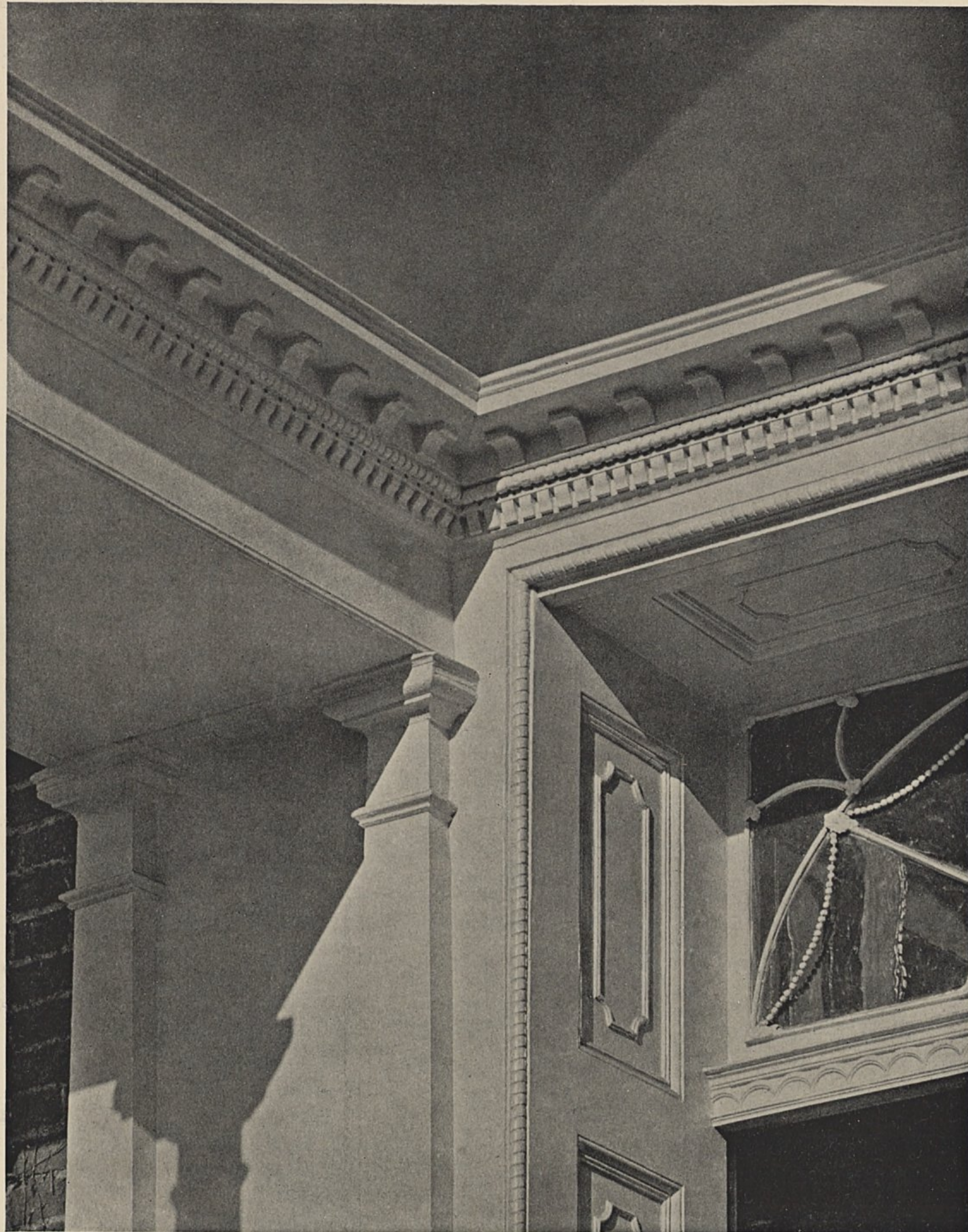
Detail of Front Porch
