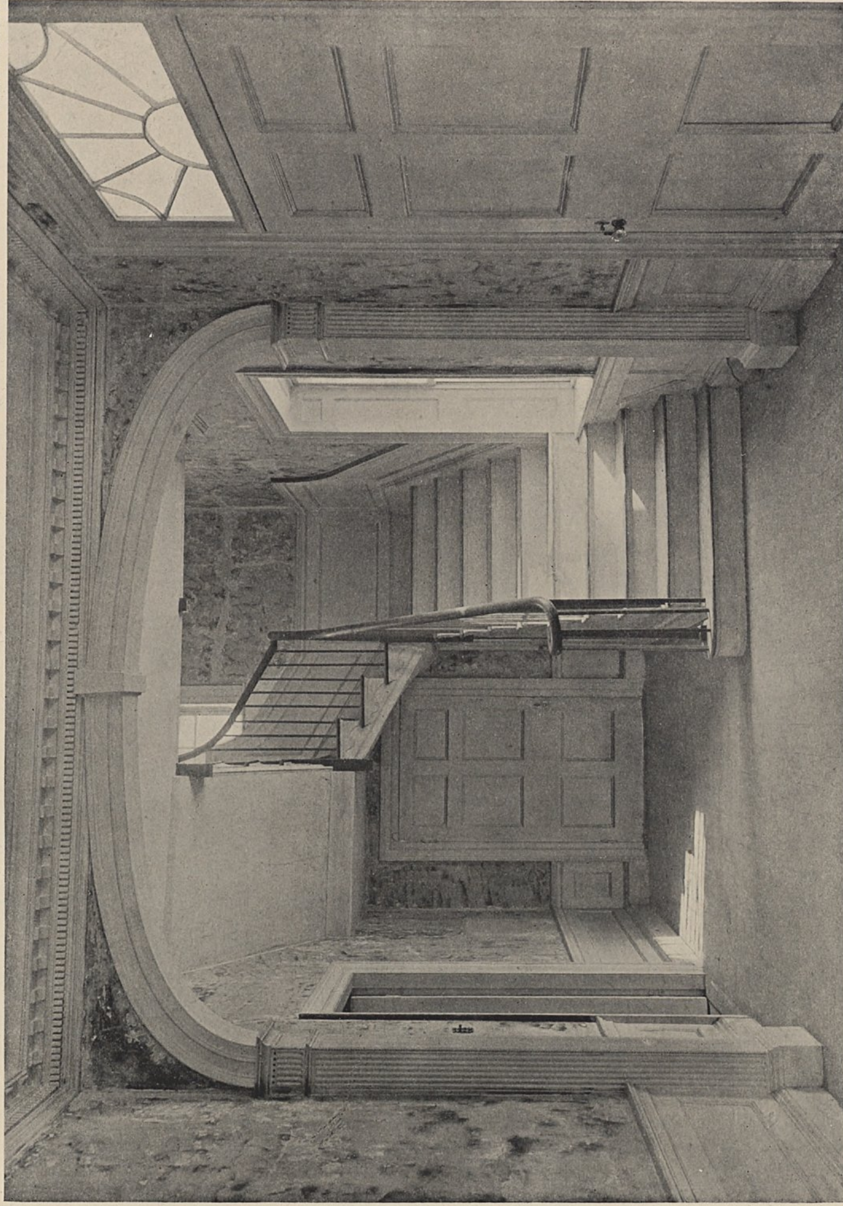
FIRST FLOOR HALL—THE SMALLWOOD—JONES HOUSE, NEW BERN, NORTH CAROLINA [Measured Drawings of the stair, published in Volume xiii, Number 2 ]
