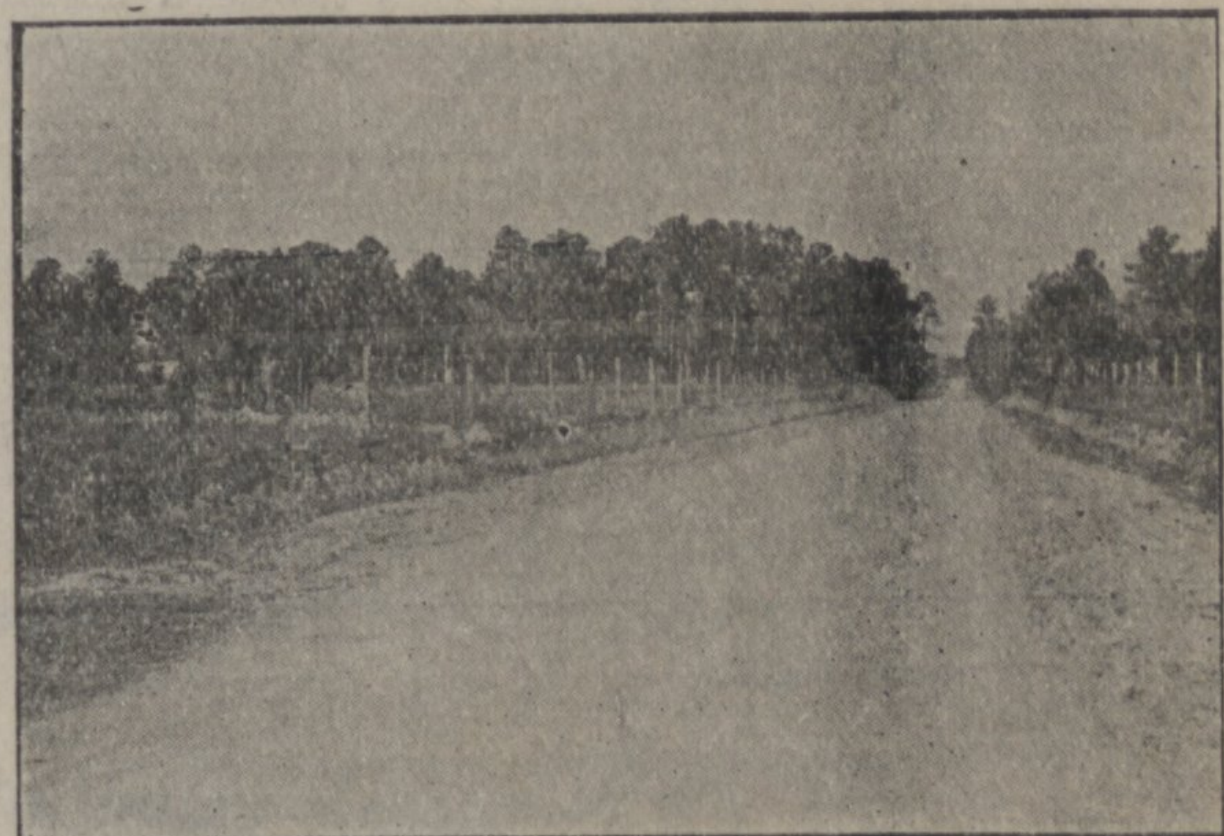
Paved Highway—Eastern Carolina
