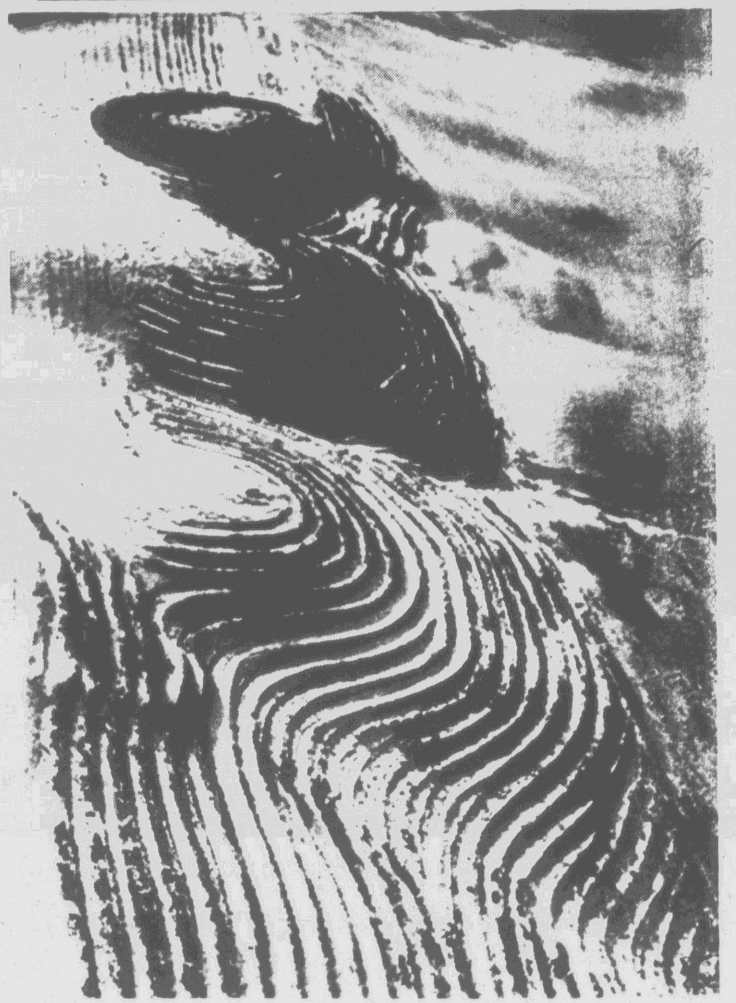
LANDSLIDE PROTECTION — Hills with terraced steps cut into them guard against landslides in the Republic of Moldavia in the Soviet Union. The official Soviet news agency Tass, which distributed this photo, said slides annually destroyed thousands of acres of fertile soil before conservation projects were begun. (AP Laserphoto)
