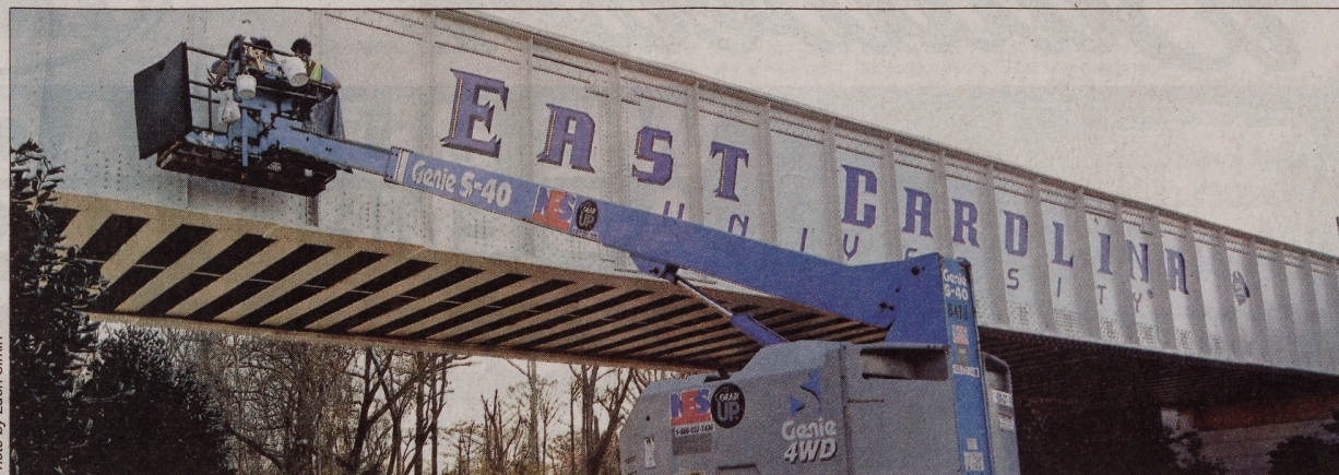
Saffo Contractors' crew works on painting Pirate logos and the words "East Carolina University" on the trestle over Charles Boulevard.
