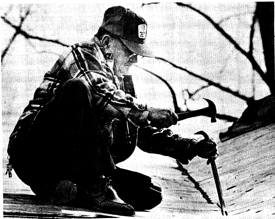
Worker renovating the roof at the Afro-American Cultural Center. Photo by Brian Hotter.
