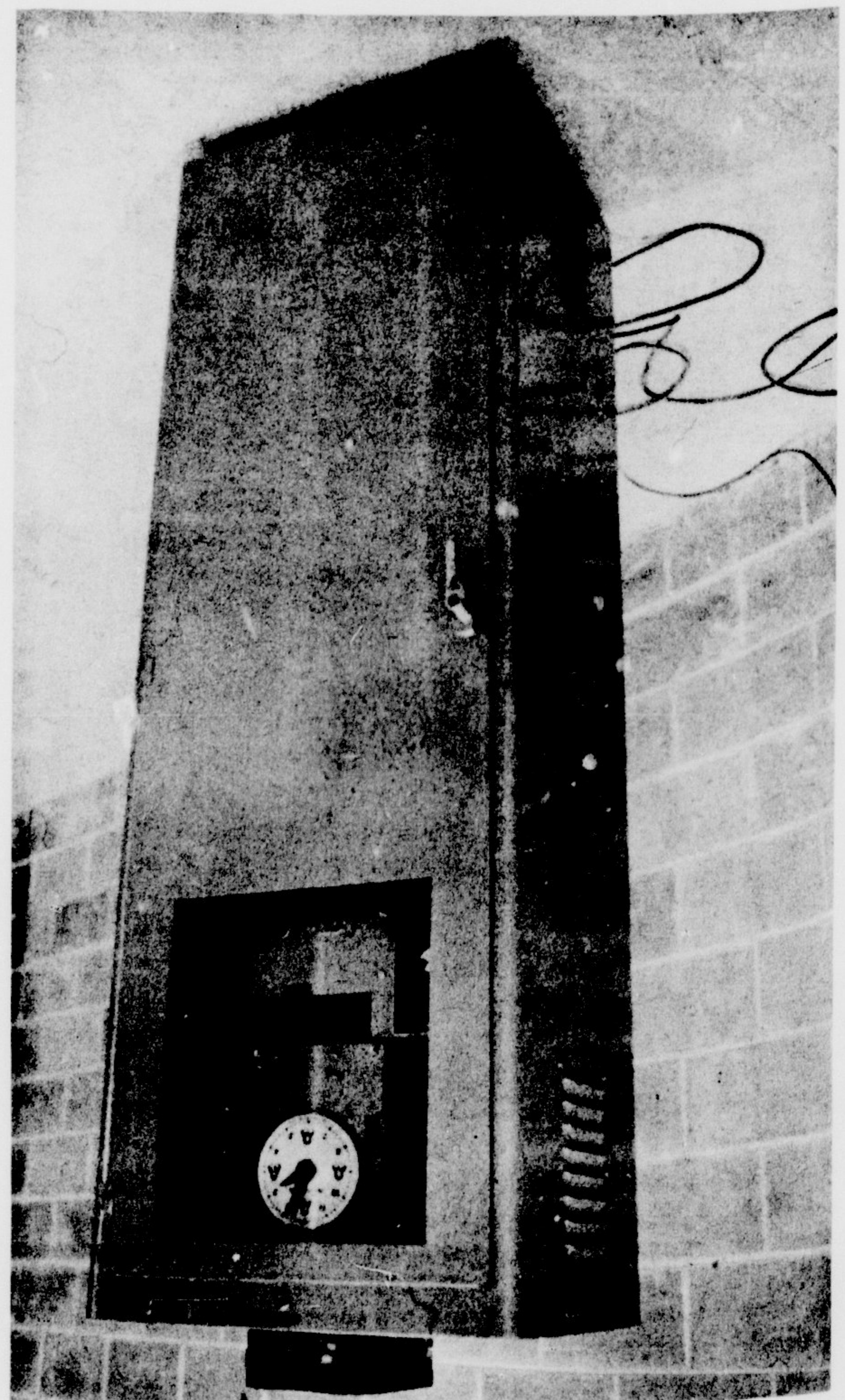
Even Chimes have brains! This is the control unit of the chimes.
