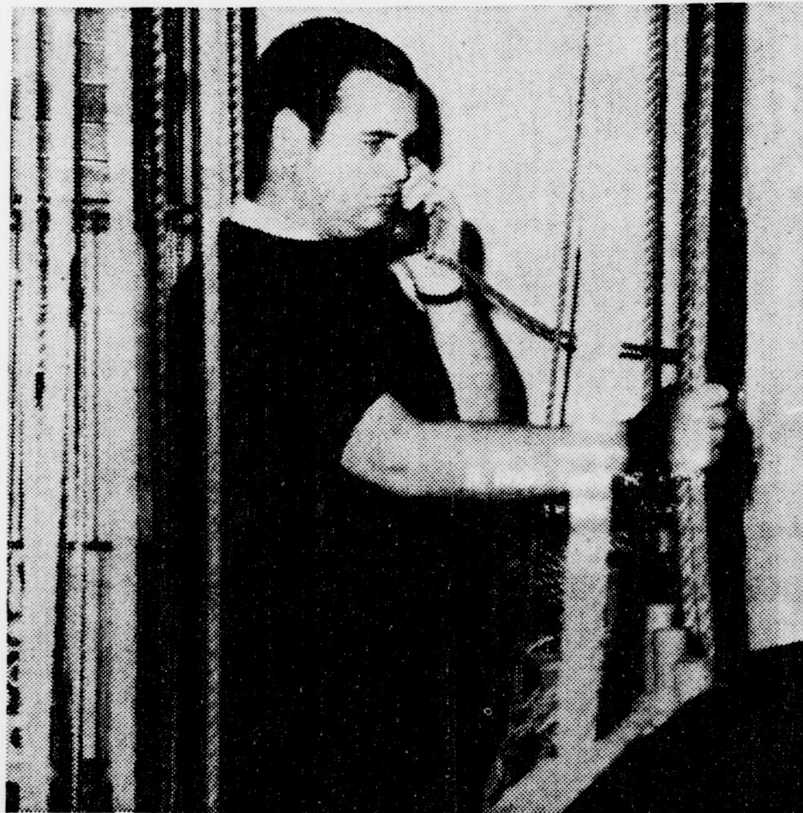
Shown here is the fly loft which the fly area space is controlled. This and the other technical stations of the play area connect by telephone.
