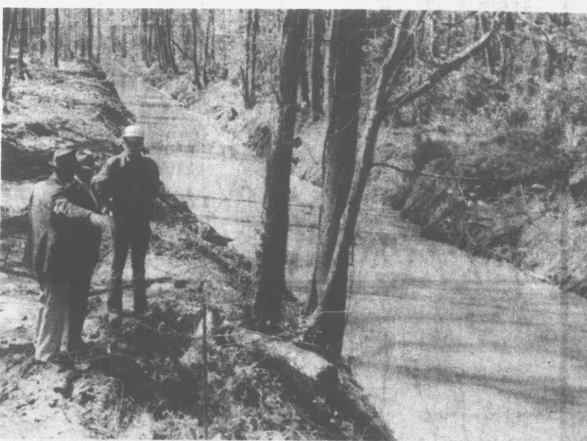
LOOKING IT OVER — Members of the Pitt County Drainage District No. 3 look over Fork Swamp Main Tuesday as the commissioners inspected
