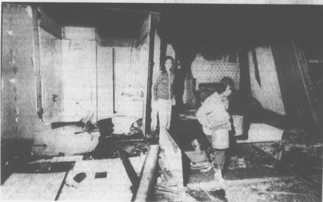
TOTAL DESTRUCTION — This is one of the many demolished homes in Wichita Falls, Texas, after a deadly tornado struck, killing at least 33 persons.
