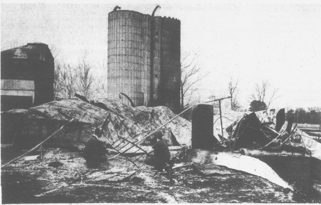
FIRE . . . left only two concrete silos at the Greenhill Dairy near here this morning. The barn and milking room and milking equipment were destroyed during the night. Vernon "Tad" Best Jr. (left) and Taylor Mosier survey the ruins. (Reflector Photo By Tommy Forrest)
