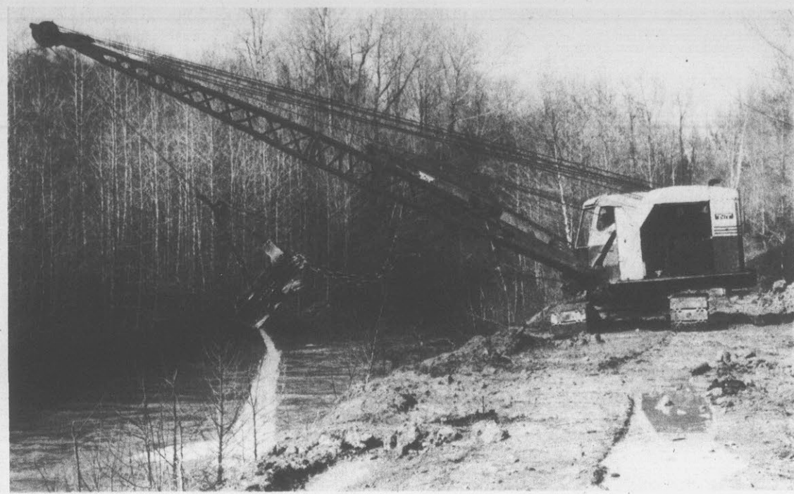
SCOOPING IT UP — Work began yesterday on the Swift Creek Watershed Project near Coxville. The first phase of the flood control and soil and water
