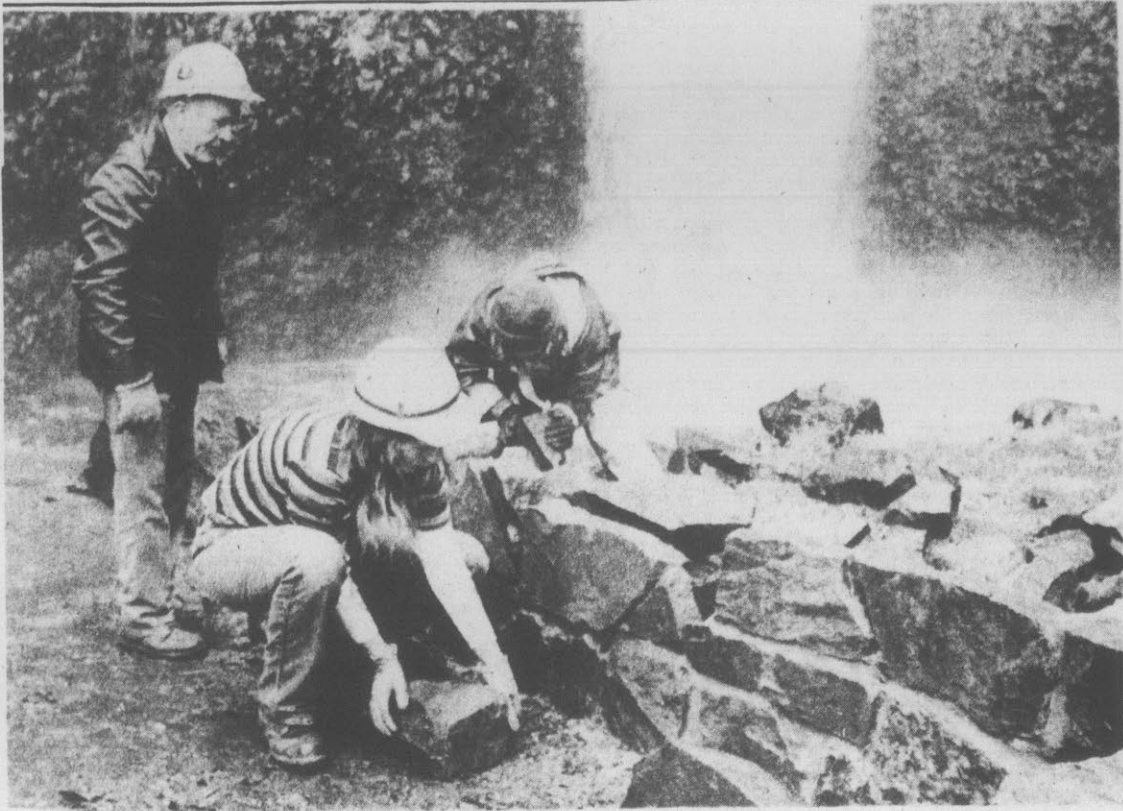
REPAIR JOB — Elmer Ayles of the U.S. Forest Service supervises repair of a rock wall done by members of the new Young Adult Conservation
