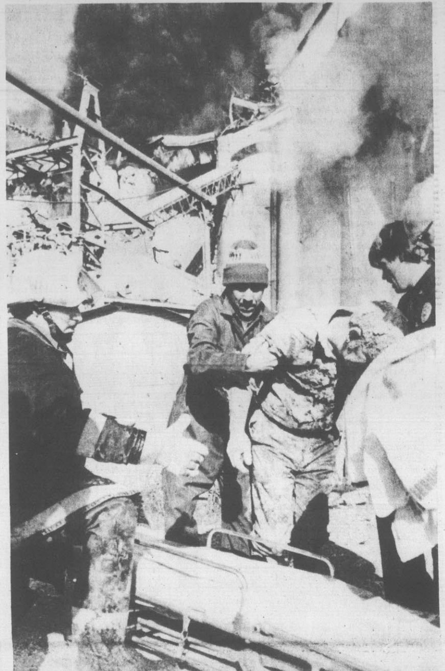
INJURED, BUT ALIVE — An injured man covered with grain dust is helped by hand with chunks of concrete passing along a human chain.
