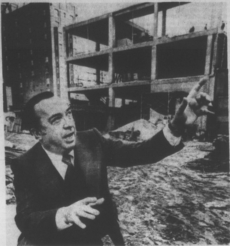
MAYOR JOSEPH LAZAROW makes a point at construction site where Resorts International is expected to open the first legal gambling casino in New Jersey. (UPI Photo)
