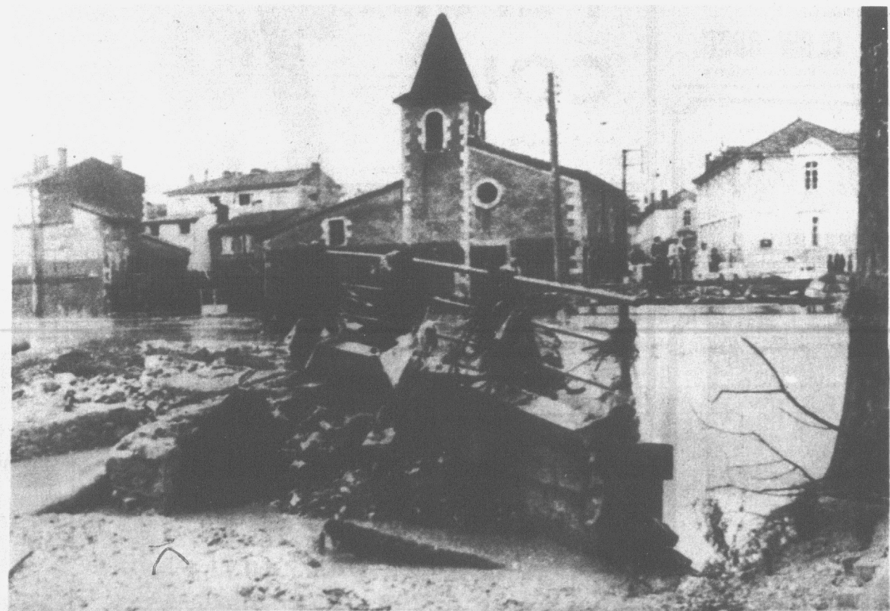
FLOOD AFTERMATH — Residents on far bank of Gers River view the remains of a bridge in Pont-Saint-Pierre, near Auch in southwestern France, Saturday, after heavy rains caused flash
