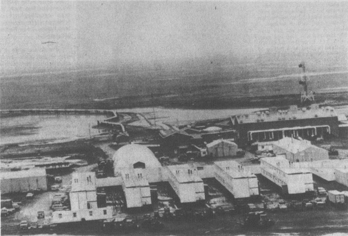
WHERE THE OIL WILL START — This is a view of Pump Station One where the oil from British Petroleum and ARCO wells merge into the Alyeska
