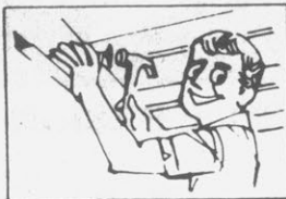
Nail up wall angles.
