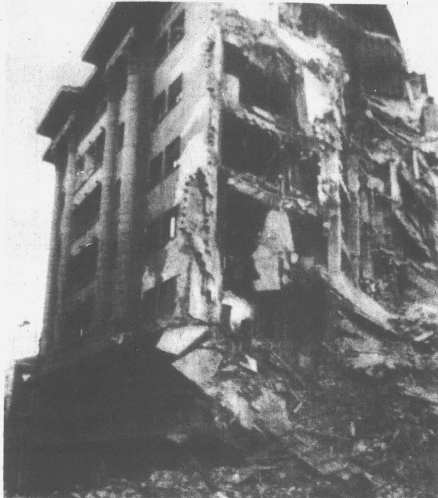
SEARCH DEBRIS — Debris lies strewn in the streets in downtown Bucharest Saturday as people search through ruins caused by heavy earthquake Friday night. Western sources estimated
