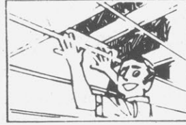
Lay in panels.
