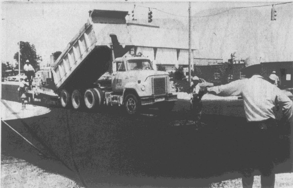
STREETS RESURFACED —City street department crews work paving streets in downtown Greenville. Streets paved include Cotanche, Third, Fourth, and Greene. Other streets are planned for the future resurfacing. According to C. A. Holliday, city engineer, approximately 1,565 tons of asphalt were used for the job, costing
